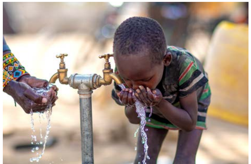
Water is stored in the tank on the tower and provides ample water without pumping by hand.
